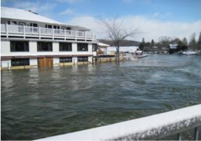
Picture taken between the 5th and the 9th of April 2014 showing the Massawippi River rising above the level of the Pilsen's ground floor.
